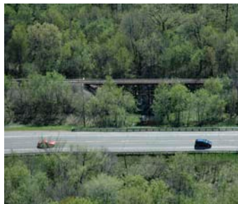
County Road 81 and BNSF Railroad over Rush Creek.
